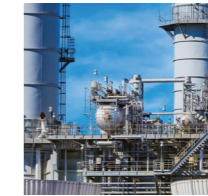
Refineries (gas compressors, gearbox)
