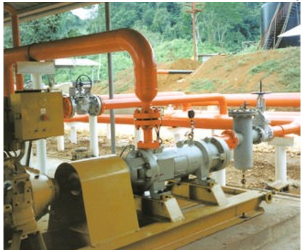
Figure 8 – Diesel Driven 3-Screw Pump at 1400 psi
