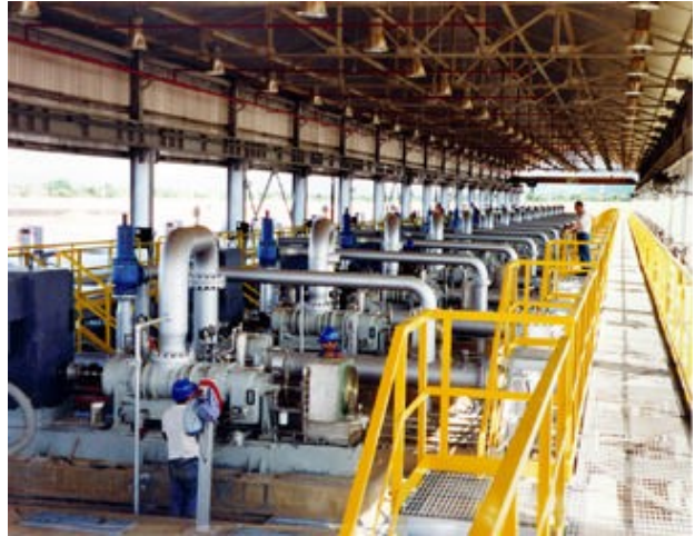
Figure 7 – 15 Twin Screw Pumps for SUBSEA Pipeline
