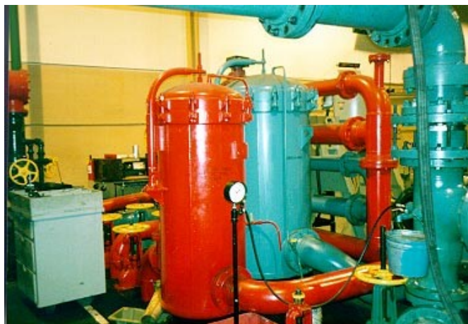
Figure 5 Single Type, Permanent Strainers
