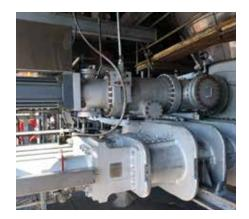
The introduction of DeltaValve's fully automated coke drum unheading valve in 2001 necessitated the development of side feed entry into the coke drum. No longer was it possible to feed resid into the coke drum through the bottom flange as was standard with traditional manual or semi-automated unheading systems.
