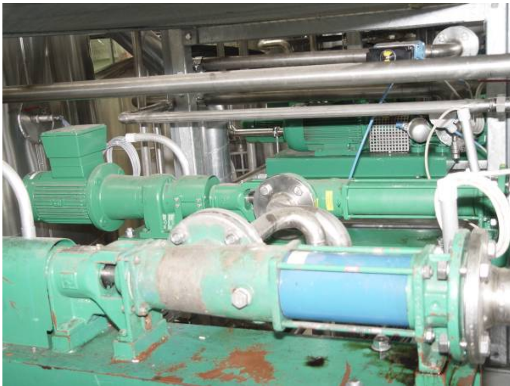
ALLWEILER progressing cavity pump for moving glycerin phase, discharge pressure 2 bar, capacity 6 m 3 /h.
