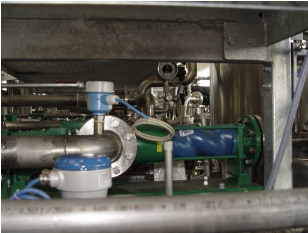
ALLWEILER progressing cavity pump for moving glycerin phase, discharge pressure 2 bar, capacity 6 m 3 /h.
