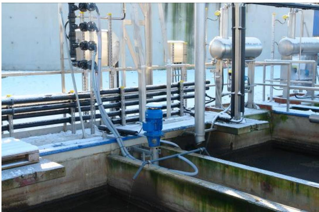
Caption: Allweiler propeller pump ("PT 300" series) for circulation (400 m<sup>3</sup>/h with 1.1 kW power requirement)
