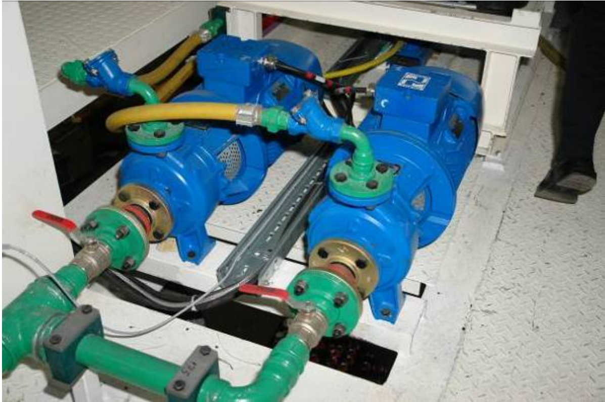
Allweiler centrifugal pumps of the “NB” series, used as water pumps.
