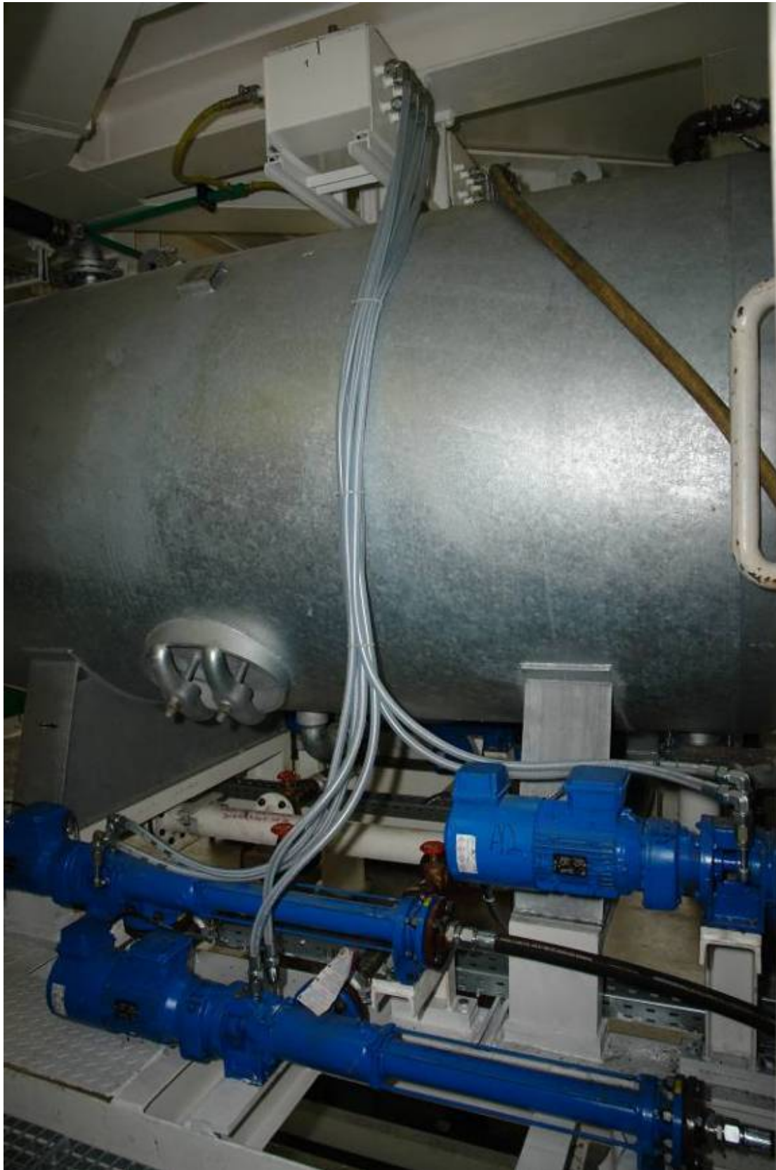
Allweiler progressing cavity pumps of the “AEB-H” series, used as proportioning pumps with a quench for accelerator.
