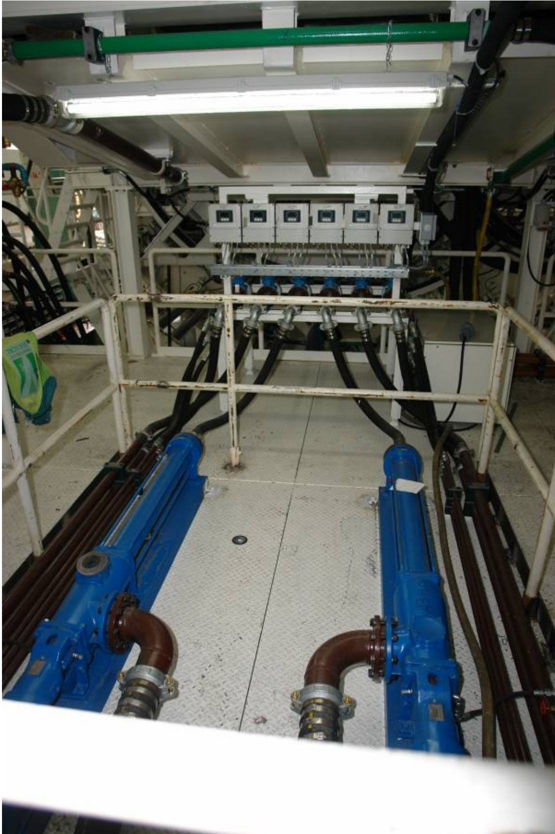
Allweiler progressing cavity pump of the “AE-H” series, used as bentonite pumps for injecting the ring-gap mortar.
