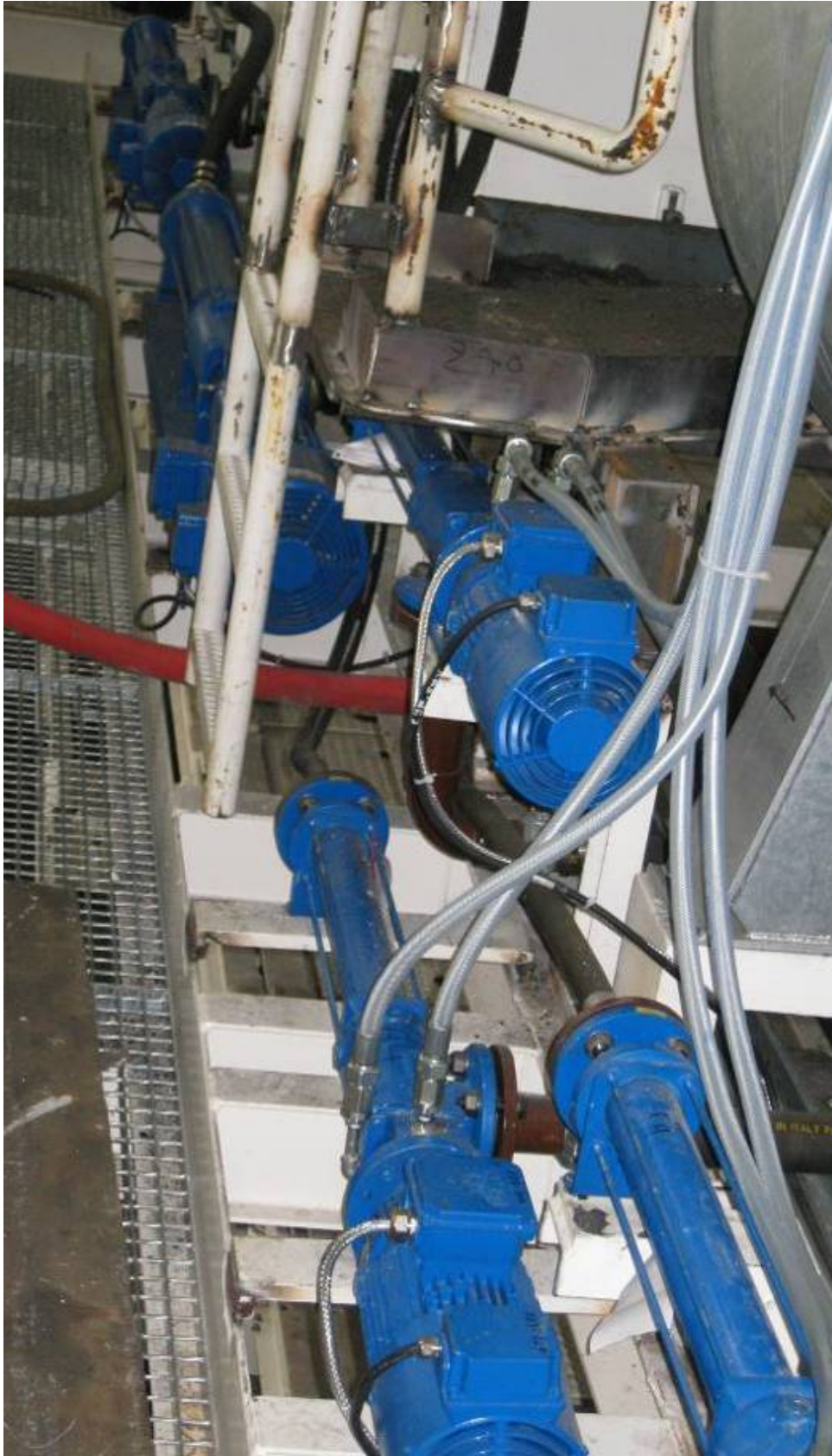
Allweiler progressing cavity pumps of the “AEB-H” series, used as proportioning pumps with quench.
