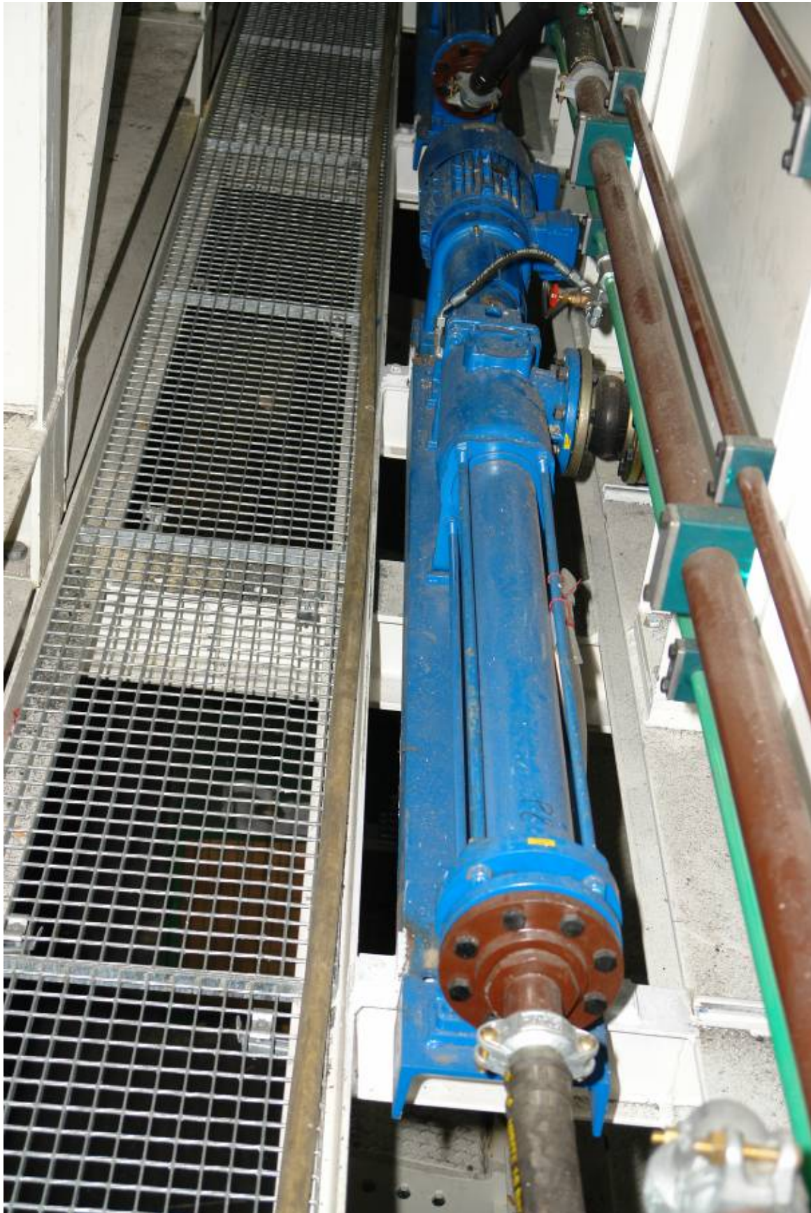
Allweiler progressing cavity pump of the “AE-H” series, used as a bentonite pump.
