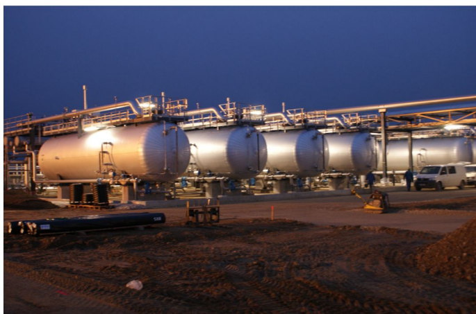
Allweiler pumps are used exclusively in the central Matzen extraction station.
