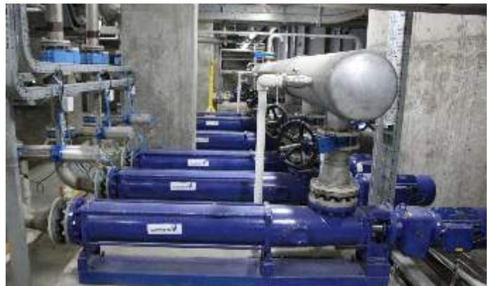
Application: Pumping sludge Pump series: ALL-OPTIFLOW® Flow: 100-150 m 3 /h / 440-661 gpm Pressure: 3-4 bar / 43.5-58 psi
