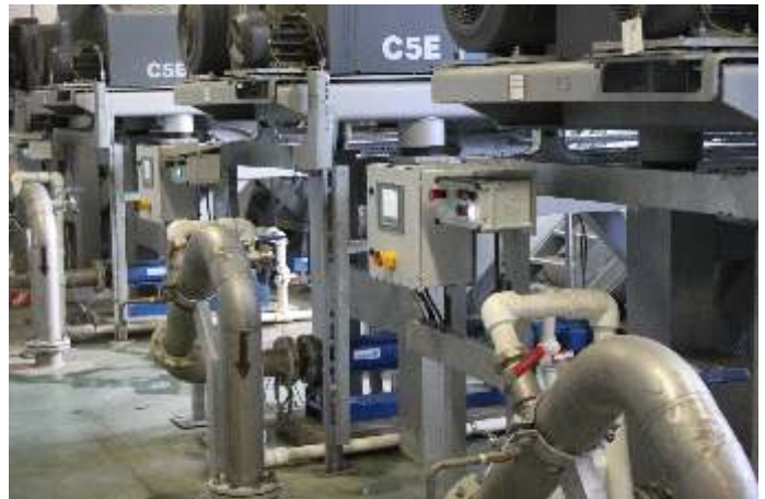
Application: Pumping thickened sludge to storage tank of centrifuges for dewatering up to 20-25%. Pump series: ALL-OPTIFLOW®
