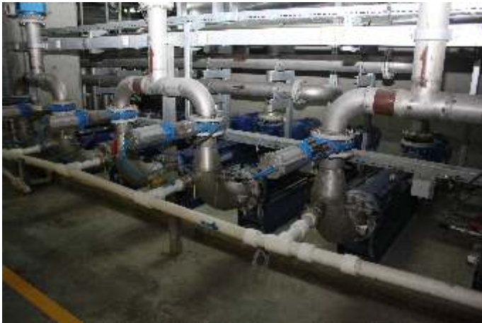
Application: Pumping thickened sludge to digesters Pump series: ALL-OPTIFLOW®
