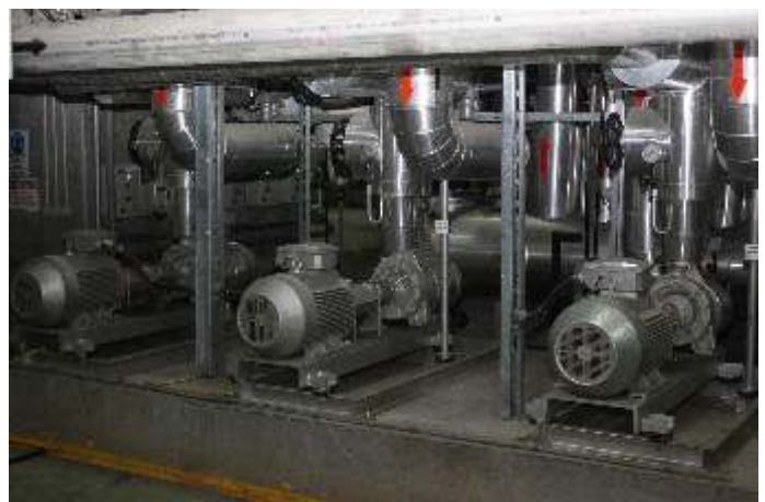
Application: Heat transfer Pump series: ALLHEAT® Temperature: 220 °C / 428 °F Pressure: 6 bar / 87 psi
