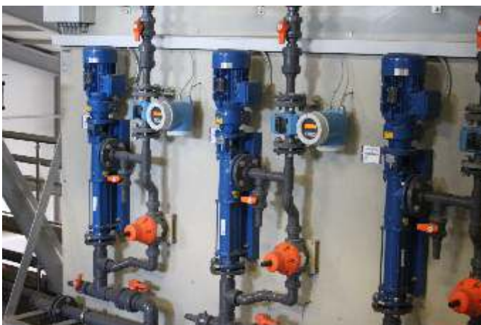
Application: Proportioning additives Pump series: ANBP
