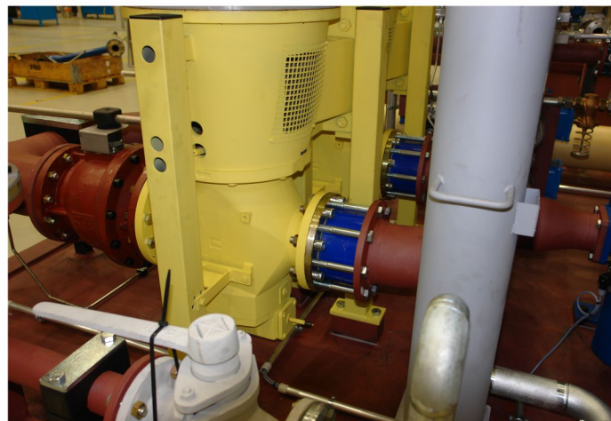
Three-screw pump of the TRF series in an oil-supply system ("OWGM" construction type) for a vertical mill drive. The pump moves synthetic or mineral oil VG320 at a pressure of 10 bar.
