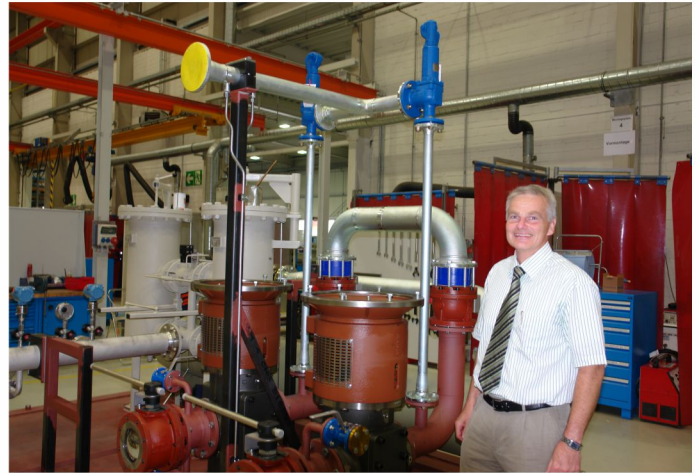
Redundant twin three-screw pumps of the SNS series in an oil-supply system (“OWGX” construction type) for an extruder drive. The pumps move synthetic or mineral oil VG320 at a pressure of 8 bar.
