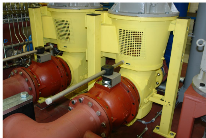
Three-screw pump of the TRF series in an oil-supply system ("OWGM" construction type) for a vertical mill drive. The pump moves synthetic or mineral oil VG320 at a pressure of 10 bar.
