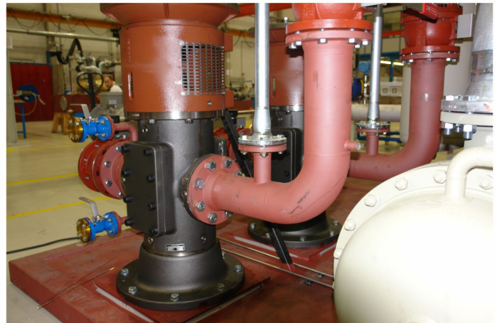
Redundant twin three-screw pumps of the SNS series in an oil-supply system (“OWGX” construction type) for an extruder drive. The pumps move synthetic or mineral oil VG320 at a pressure of 8 bar.
