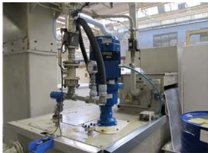
Electronic control with a frequency converter in a remote switch cabinet, after conversion.
