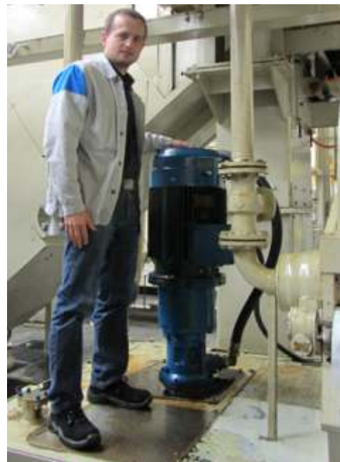
"The conversion allows us to process about 200 more transmissions each month. Aside from the energy savings, this is a critical point for us," according to Dipl.-Ing. Jan Wettlaufer, technical manager in housing production. Image shows one of the electronically controlled EMTEC screw pumps.
