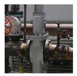
The GV851 is a high performance isolation gate valve specifically designed for clean services within the delayed coker. Such services include steam and water, clean hydrocarbon liquids below coking temperatures, and clean hydrocarbon vapor streams in on/off and modulating services.
