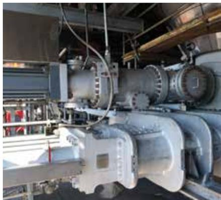
The introduction of DeltaValve's fully automated coke drum unheading valve in 2001 necessitated the development of side feed entry into the coke drum. No longer was it possible to feed resid into the coke drum through the bottom flange as was standard with traditional manual or semi-automated unheading systems.
